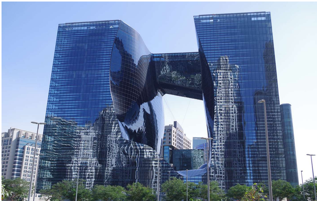
Comparison single corner cold-bending vs. free form cold-bending, incl. structural silicone stress models Benjamin Beer / Ramboll
